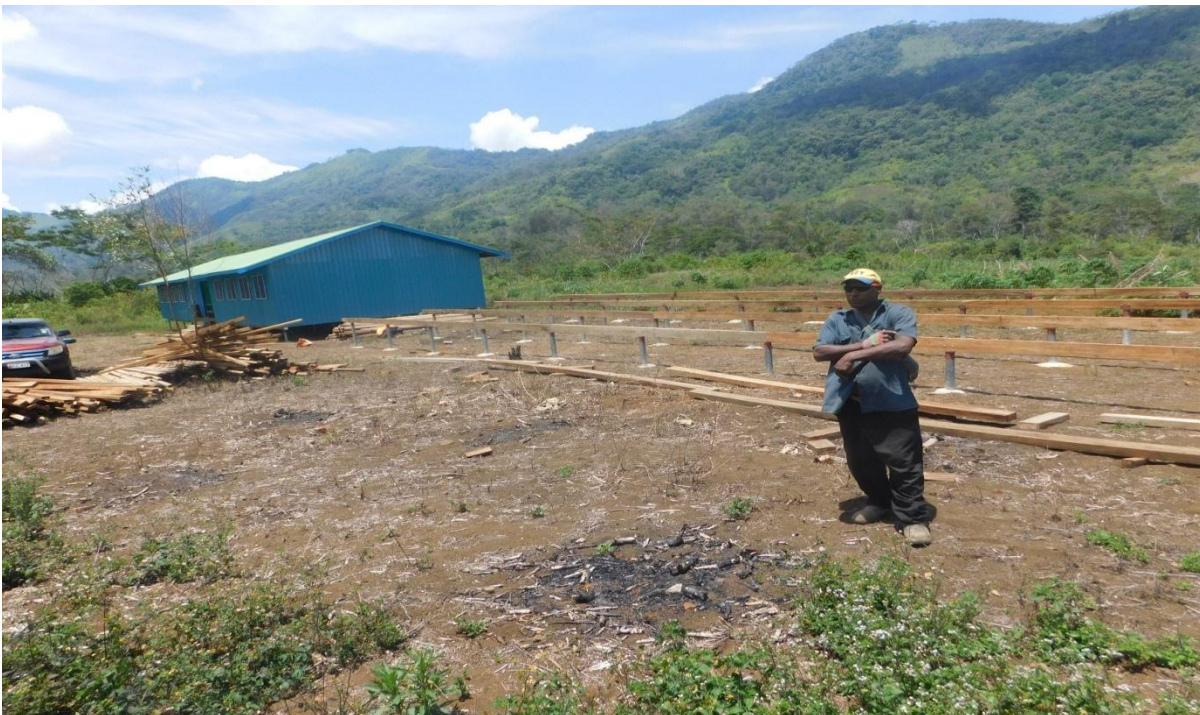
New Ukinin Maiwa Baptist High School under construction 2019-2020
