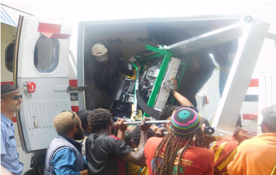
Delivery of Lucas Mill to build classroom & staff houses in Enga Baptist Union (Lapolama Primary School)
